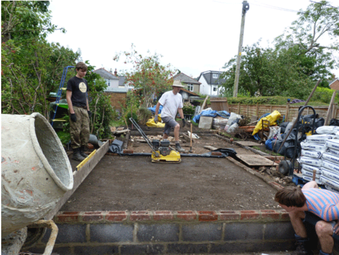
Preparations for the concrete slab at the demolished bomb shelter site.
